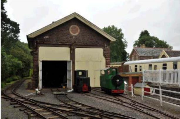
[Above] The old goods shed now the work shops for the narrow gauge railways. Note the two differing track gauges.
